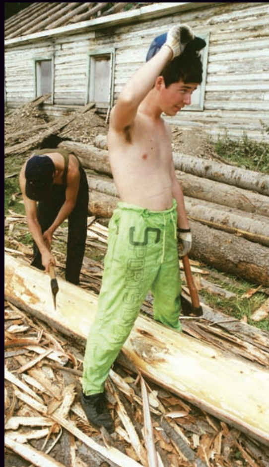
THE CAMP’S SAWMILL, BELOW, HAS BEEN PUT BACK INTO SERVICE TO PREPARE LUMBER NEEDED FOR THE RESTORATION PROJECT. VOLUNTEERS, RIGHT, REMOVE BARK FROM TIMBER BEFORE SENDING IT ON TO THE MILL.
